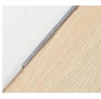
Step 1: Put a BerryAlloc Fillertwine in the expansion gap (8-10mm). The Fillertwine allows the laminate to expand/shrink. Also use a Fillertwine in the expansion gap under floor profiles such as T-profiles, reducers,...
