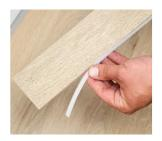
**Step 3**: Apply a HydroPlus Strip to the base of the skirting using the adhesive strip. This strip protects your skirting from water, while still allowing the laminate underneath to expand/shrink.
