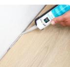
**Step 2**: Put HydroPlus Sealant on top of the Fillertwine. The Sealant should touch the wall and the laminate and be applied in a way that it completely closes the gap. With floor profiles, use sealant on top of the Fillertwine before you install the profile to avoid water contact with the side and the base of the laminate.
